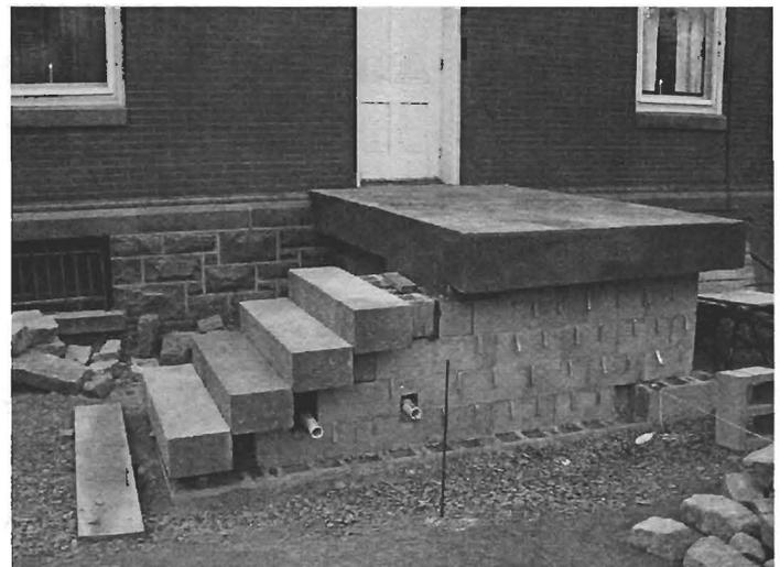
**Here The Concrete Cap Is Finished And Our Original Steps Are Being Reinstalled On The New Foundation**
